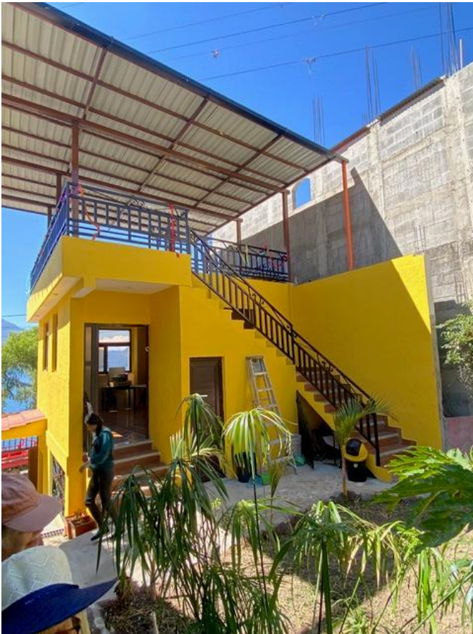
View from back of Building
