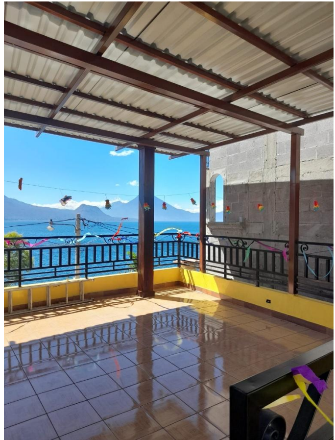
Top Floor, with view
