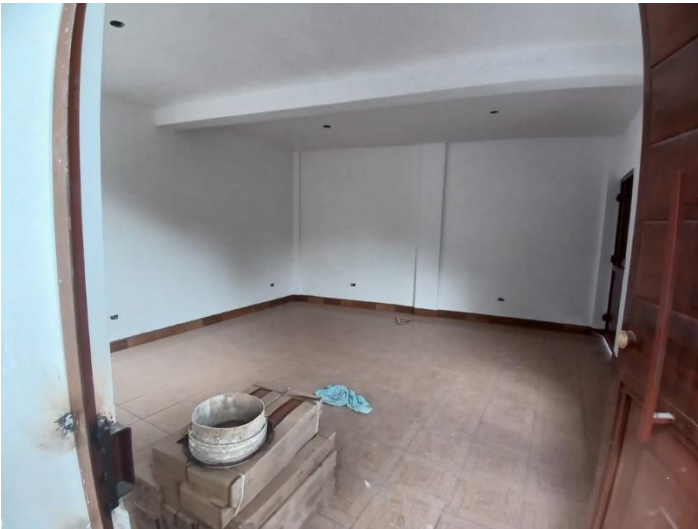
Ground floor Room
