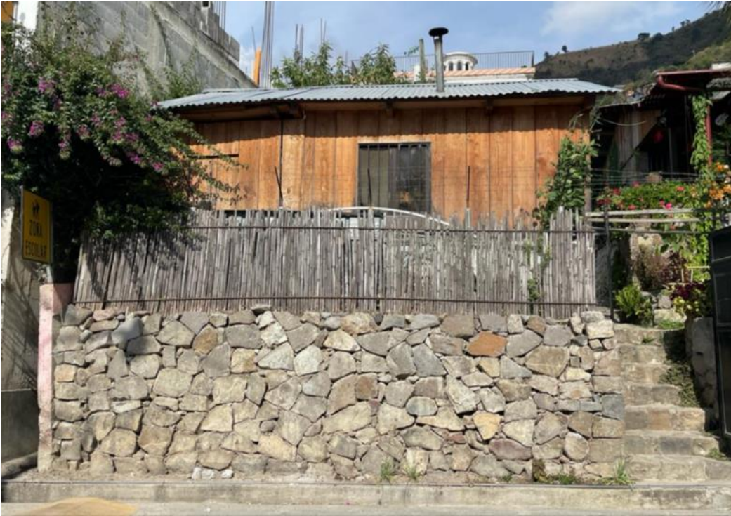
View of old kitchen building:
